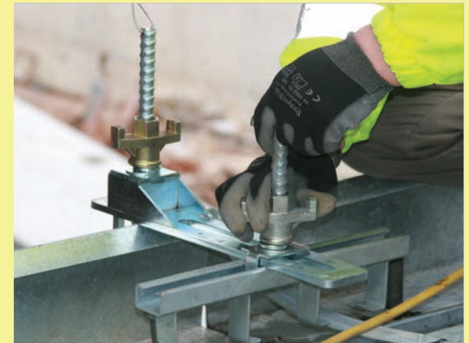
...ON A STEEL FRAME
